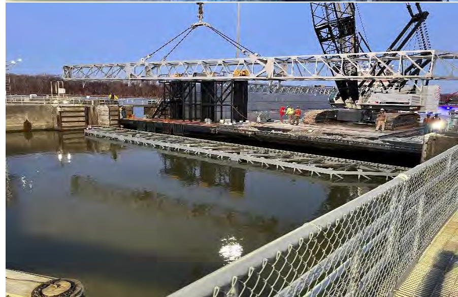
Placing Stoplogs
