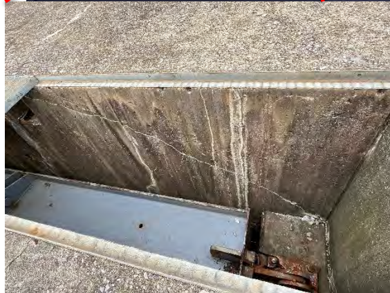
New Crack in Upstream Bulkhead Slot
