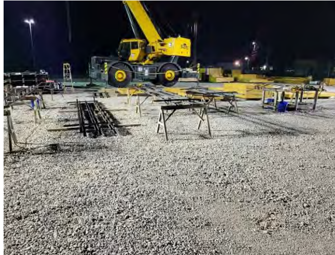
Initial Formwork Assembly
