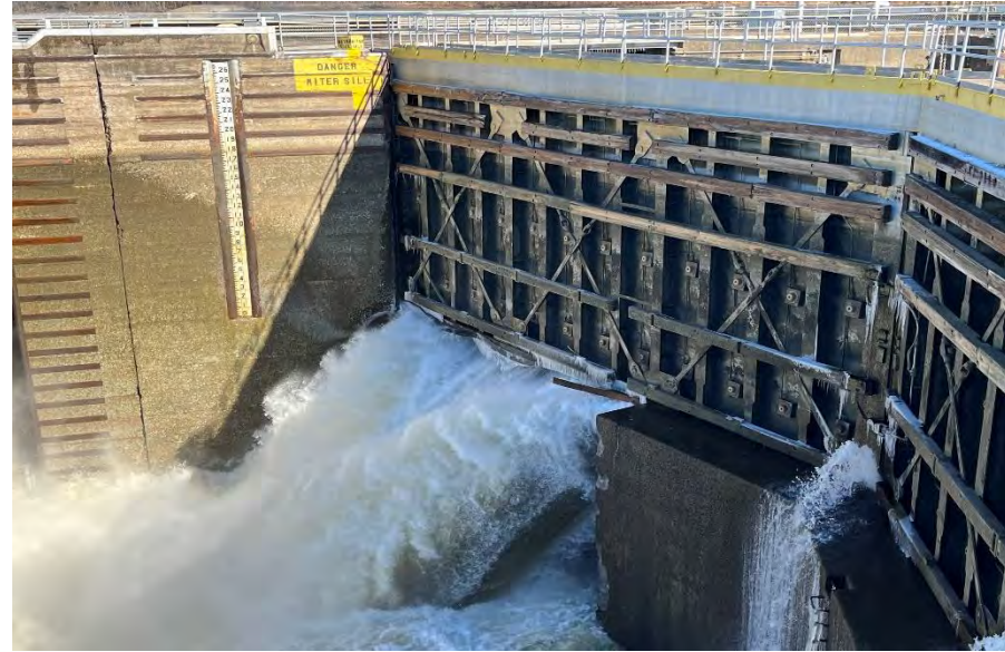
Breach Through Failed Sill
