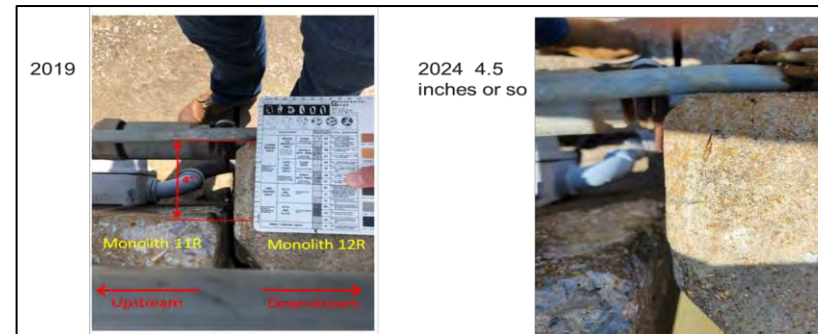
Monolith movement upstream of sill
