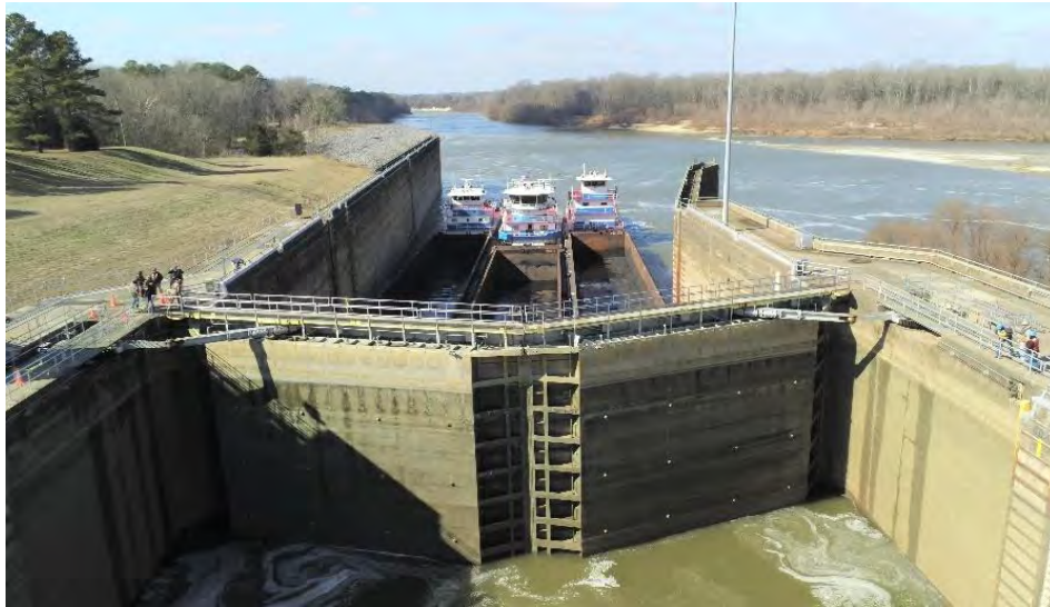
Lower Miter Gate Closure
