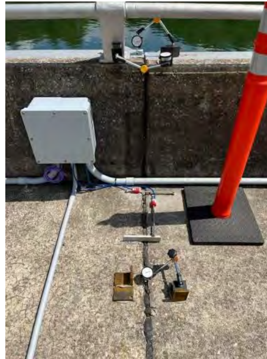
Instrumentation at Monolith Joint
