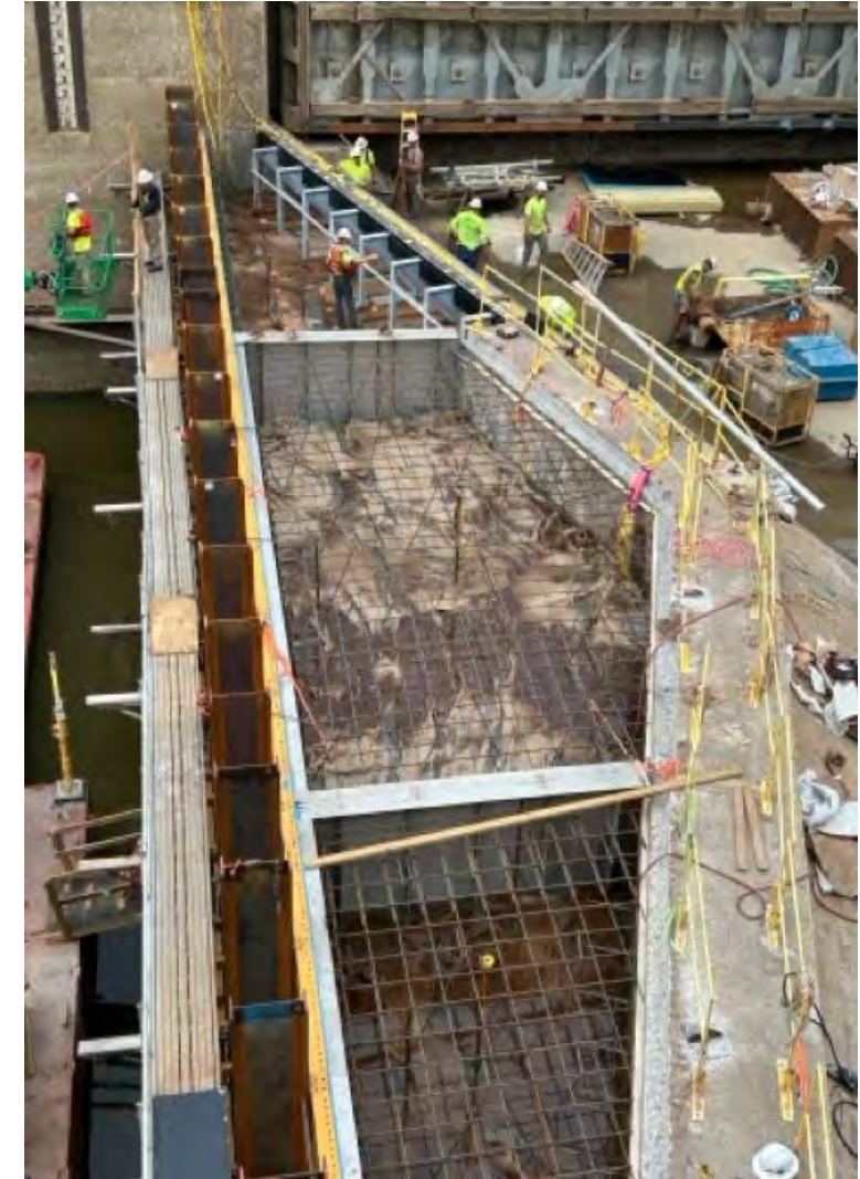
Reinforcement & Embedded Steel
